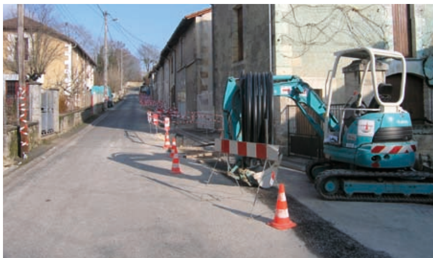
Bore path with 5 opened house connections.
