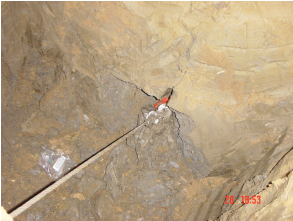
PHOTO 11 – Showing the winch cable pulling in the arriving of the GRUNDOMAT with the Front-End Expander.
