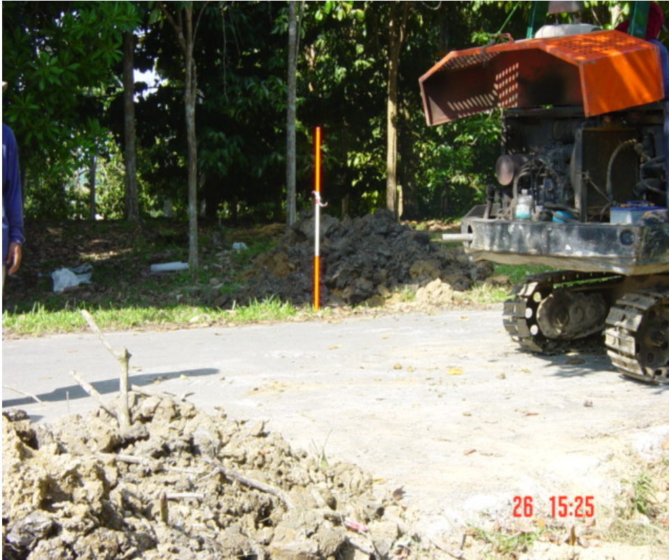
PHOTO 1 – Overall view of proposed road crossing
