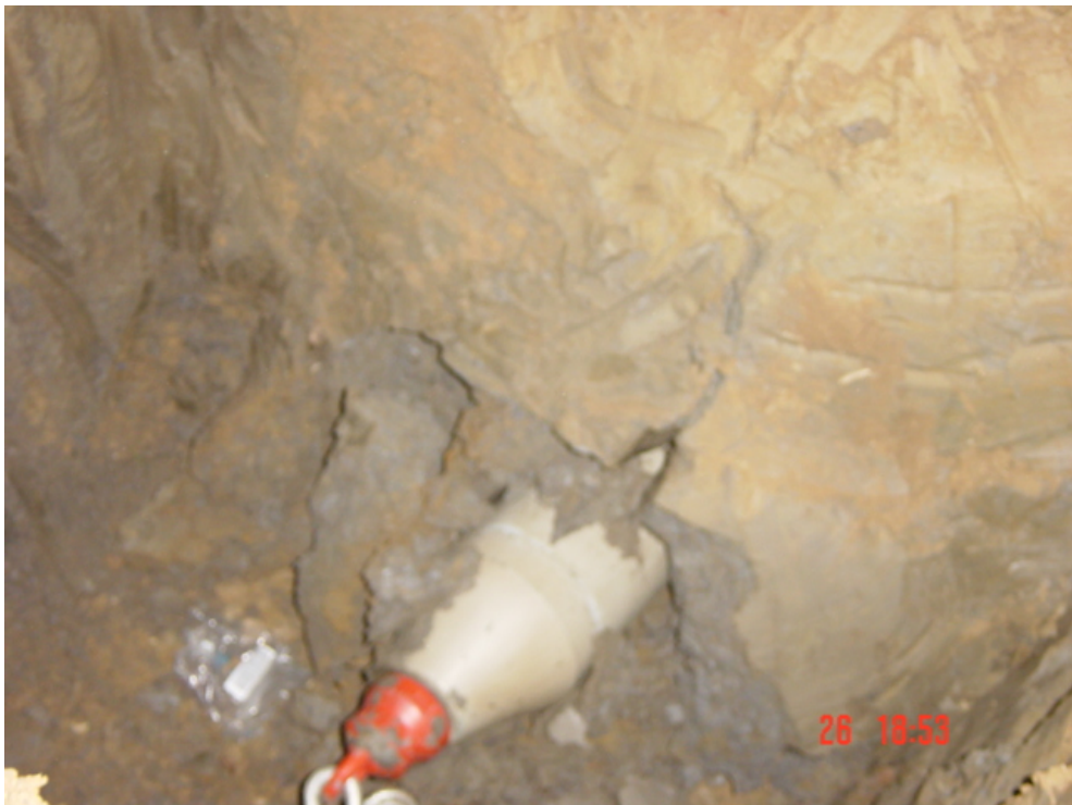
PHOTO 12 – Showing the completion of upsizing of the borehole.
