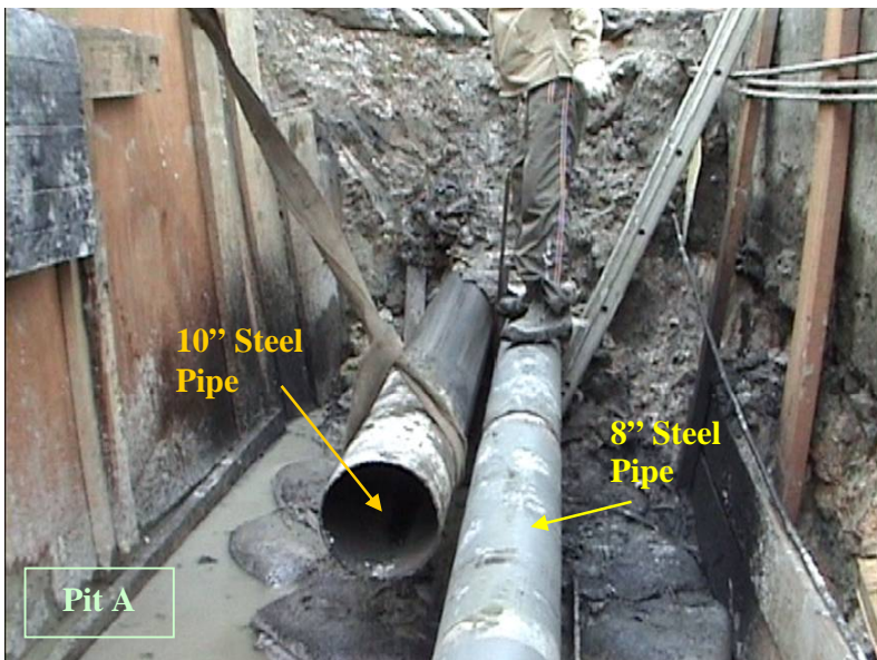
Photo 13: The old 10" Steel Pipe exit at Pit A
