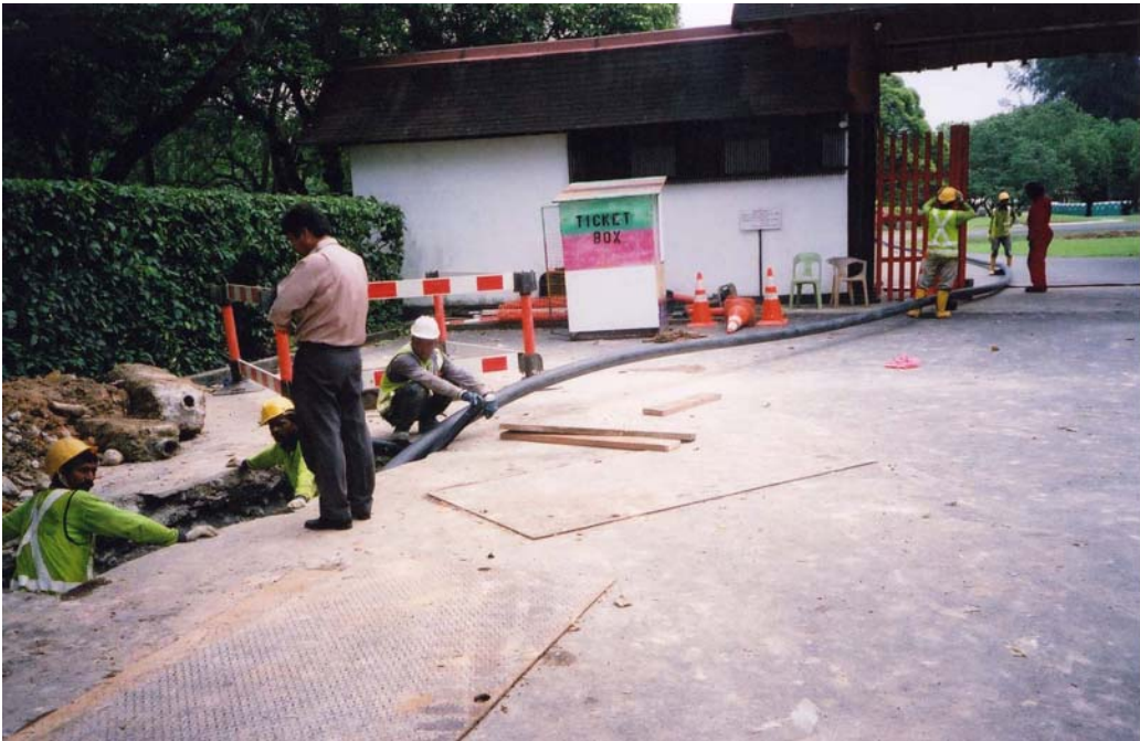
PHOTO 12 – Shows the 125mm PE pipe laid out during The bursting operation. Time taken to complete the bursting operation was 2 hours 10 minutes
