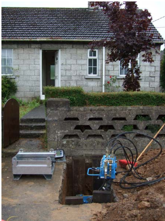
The GRUNDOPIT launch pit.
