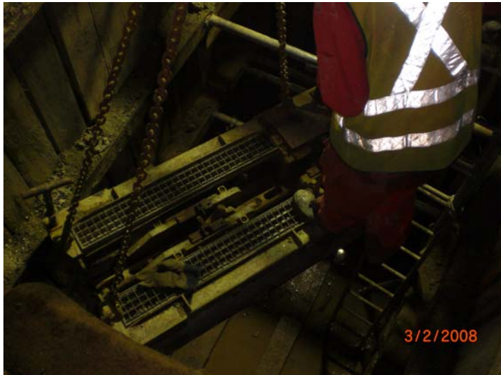
GRUNDOBURST in place to use 80 ton pull back force to pull back the pipe ready on the other side through the Quick Lock Rods.
