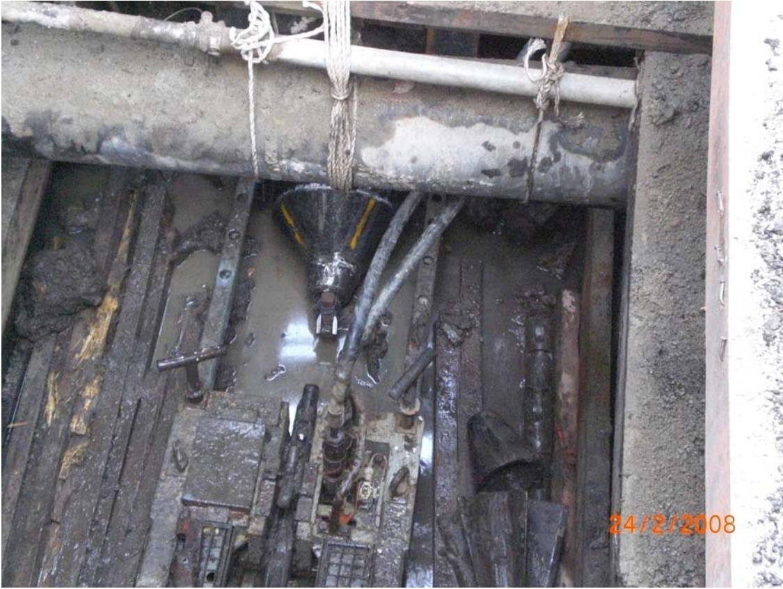
Job completed. Pipe arriving at the entry pit.
