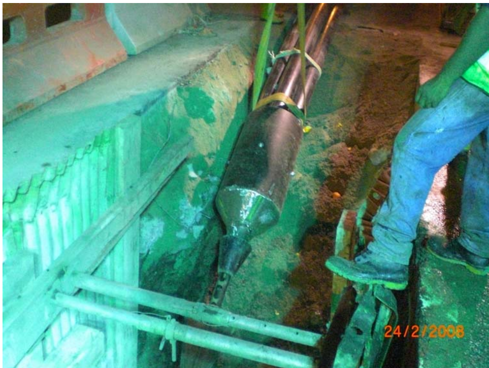
GRUNDOBURST in place to use 80 ton pull back force to pull back the pipe ready on the other side through the Quick Lock Rods.
