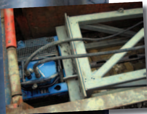
The Grundoburst 2500G rig with its extension frame in place during the Berlin swagelining operation
