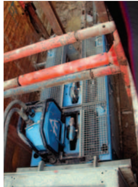
The Grundoburst 2500G in the swagelining operation
